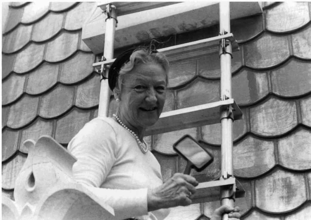
On the roof of the Shrine of the Báb, Rúḥíyyih Khánum examining the tiles for possible repair, 1977
